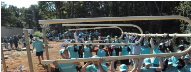
Students construct the the KaBoom! playground in Reid Park
